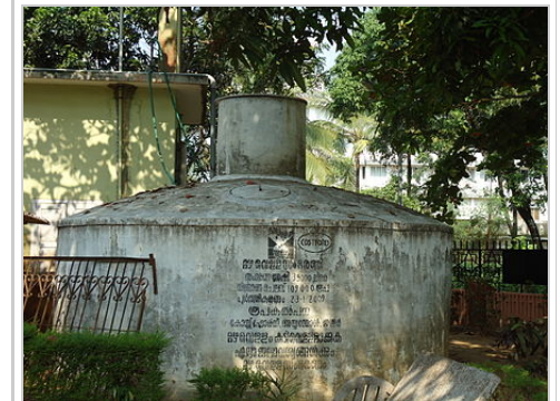
A 35,003 litre rainwater harvesting tank in Kerala
